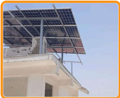
Rooftop Solar Installation
