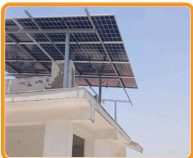
Rooftop Solar Installation
